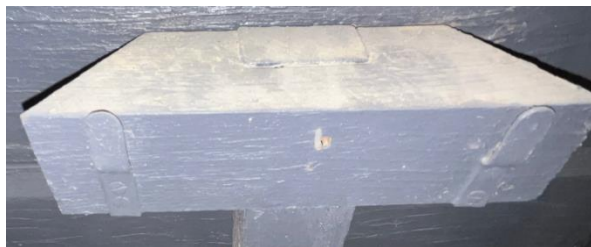
Horizontal t-mount with angle cut shown.
